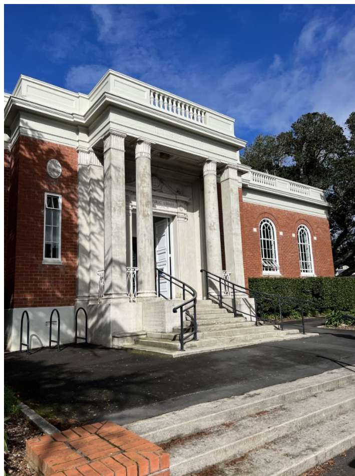
Fig. 8 – Remuera Public Library – Main Façade facing Remuera Road, 28.08.2022 Photo by Author
