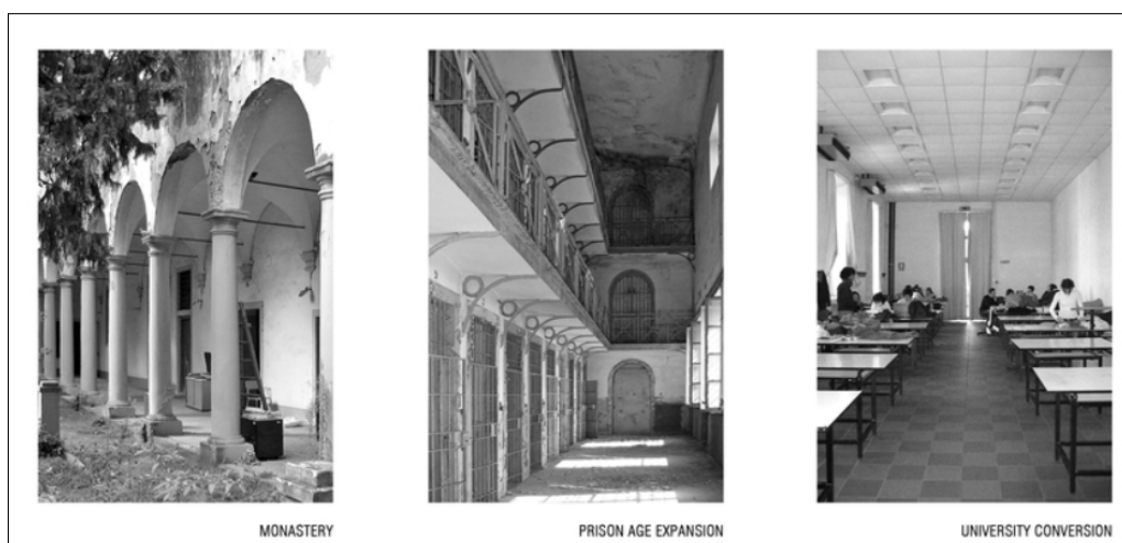
Fig. 1 – previous situation of Santa Teresa
