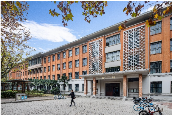
Fig. 2 – South building facade
