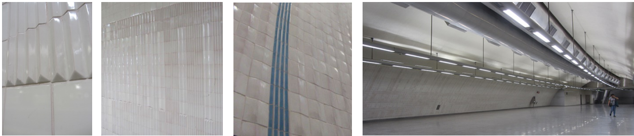
Fig.3 – Application of Maria Keil tiles in São Sebastião II station, by Catarina and Rita Almada Negreiros. Source: Margarida Gamito, 2022.
