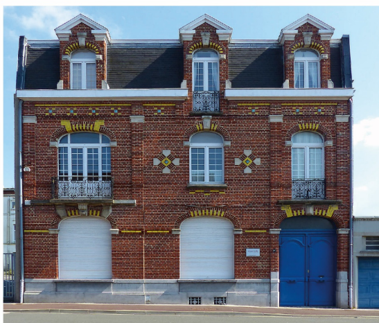
The glazed bricks on the ornate facades in Tourcoing, rue des Ursulines
