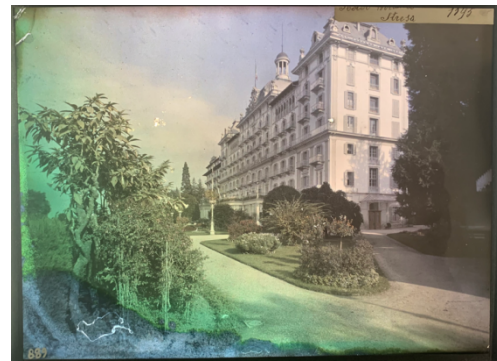
Fig. 9 - Colour bleeding and mould.
