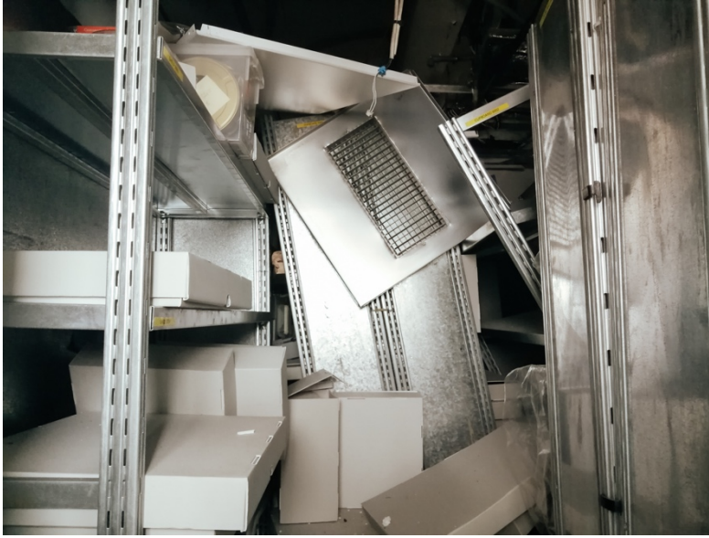
Fig. 9 The cool storage room the day after the explosion at the Beirut Port in August 2020.
