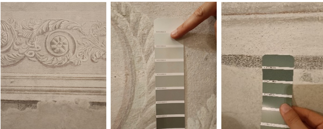
Fig. 7,8, and 9 - Visual survey of Piermarini's original decorations.
